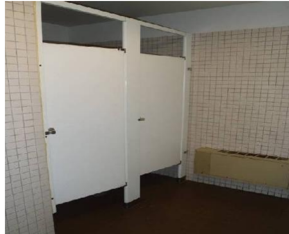
Existing Washroom / Change Room Facilities do not comply with Universal Design Requirements
