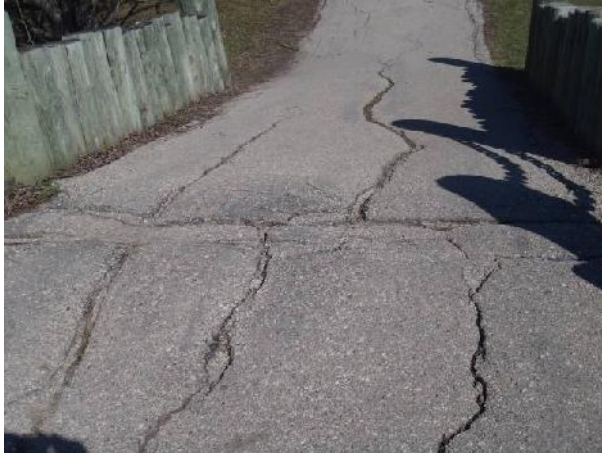
Pathway to Clubhouse from south parking lot area
