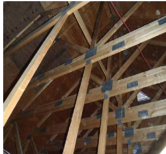
General view of roof trusses
