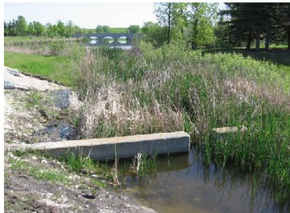
Blockage of outlet with overgrown vegetation
