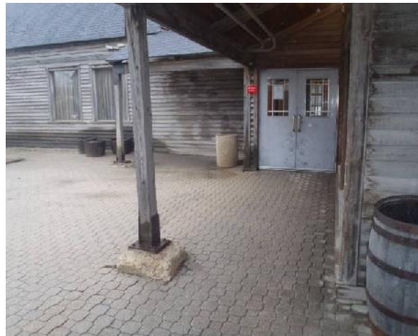
Deterioration in canopy pile cap
