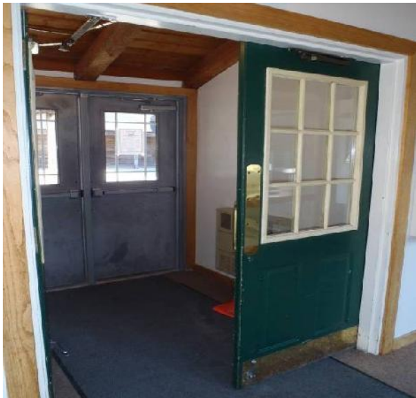
Clubhouse double exit door c/w permanent centre door mullion. Vestibule length is not in compliance with ADS
