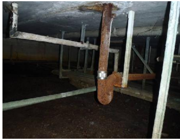
Rust on pipes and pipe hangers in the crawlspace
