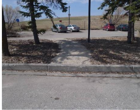
Existing Access point to H/CAP Parking Stall
