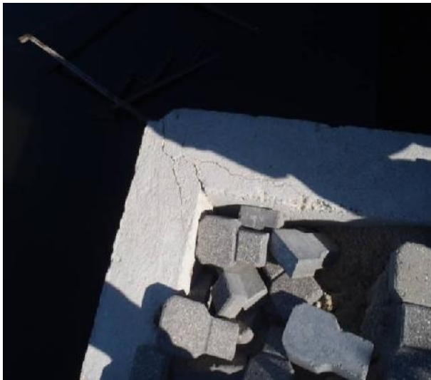
Crack at corner of retaining wall
