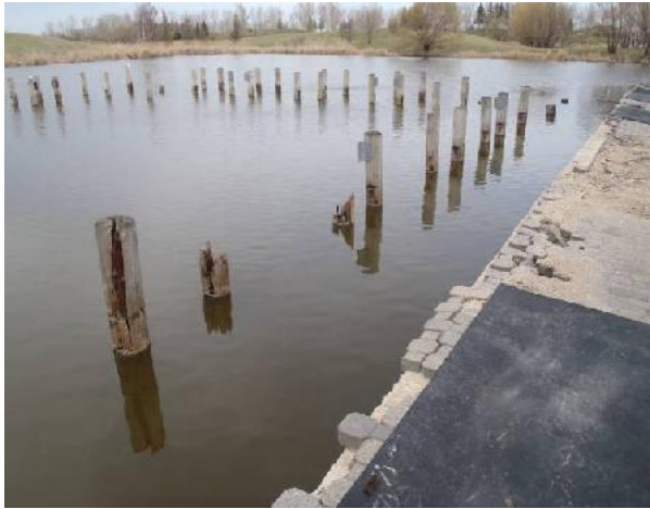
No guard rail installed along the edge of the retaining wall
