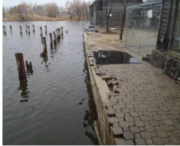
View of retaining wall along water's edge
