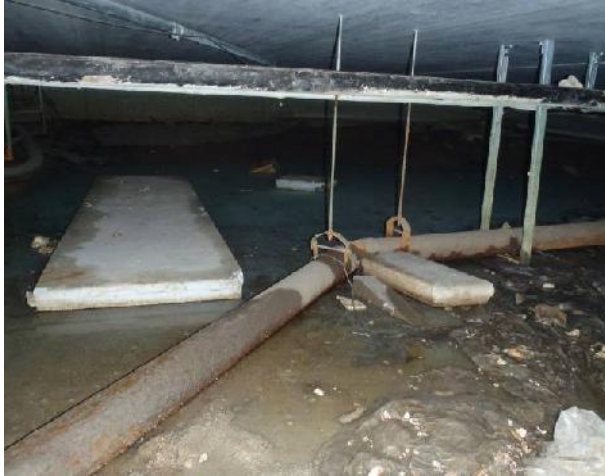
Loose rigid insulation floating on the water under the kitchen area
