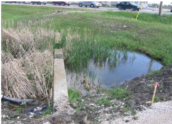
Water flowing into SRB outlet weir after May 29, 2012 event
