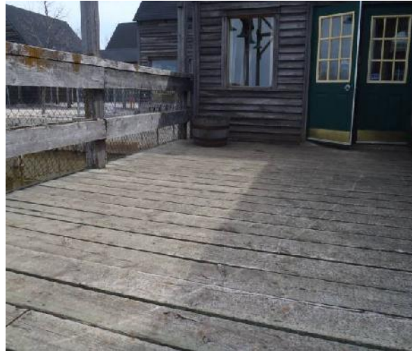
Aged deck floor and guard rail systems
