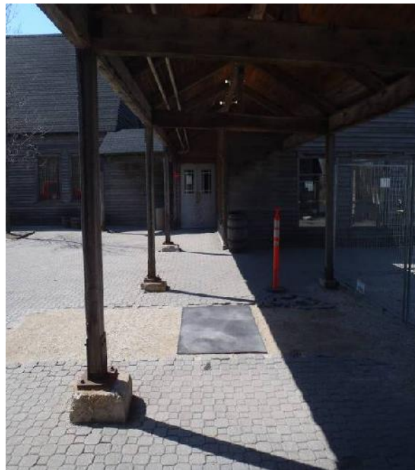
Areas of paving stones needing replacement
