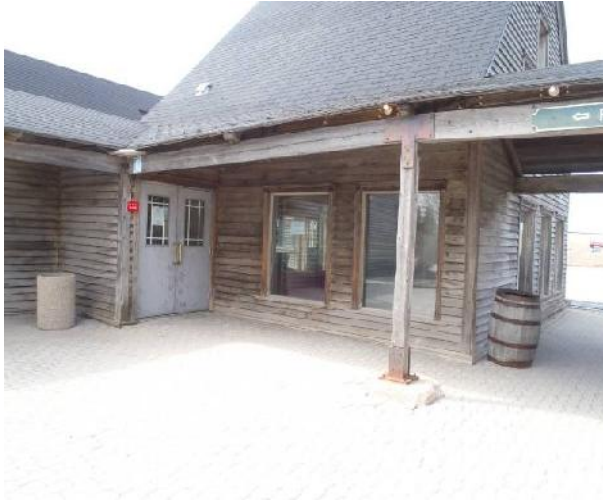
Heaving of canopy column
