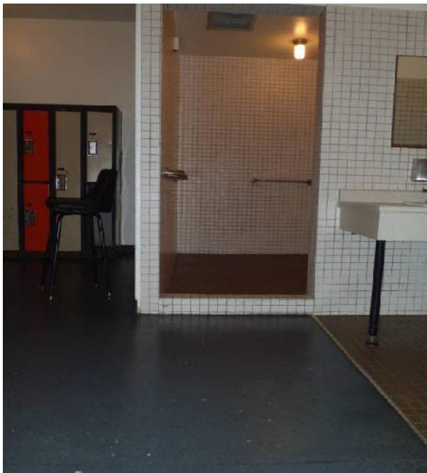
Entry into shower stall area not barrier-free
