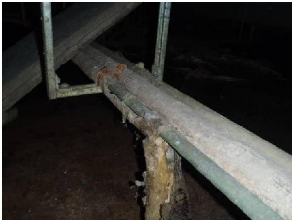
Missing insulation around the pipe
