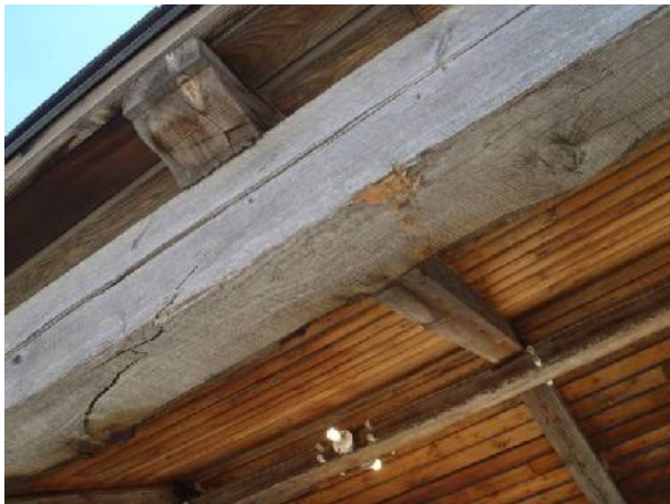
Crack in the Canopy beam
