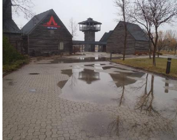
View of the main courtyard area of the Harbour View Facility
